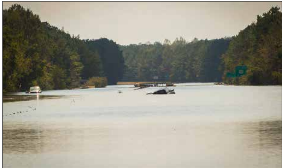
Figure 1. Interstate 40 flooding during Hurricane Florence (photo courtesy NCDOT).
