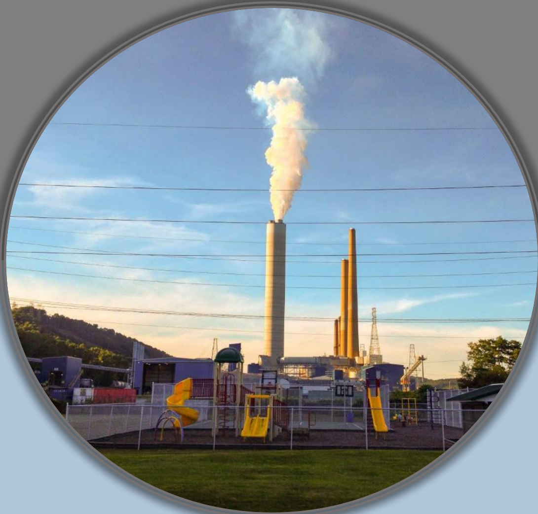
FirstEnergy's W. H. Sammis Plant, Stratton, OH
