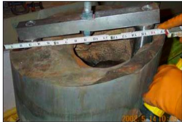
The hole in the Davis-Besse reactor head, 2002
