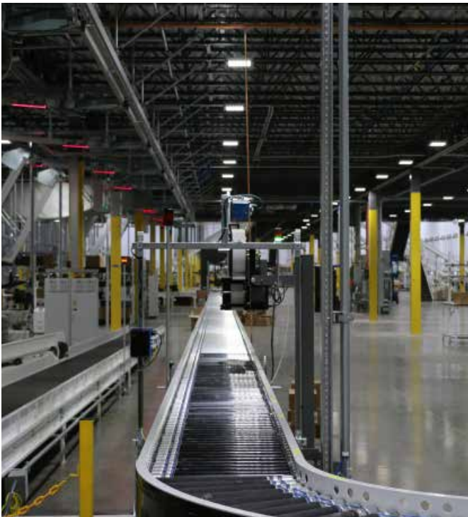
REI's 2.2 MW onsite solar system is capable of meeting all of the distribution center's annual power needs.
