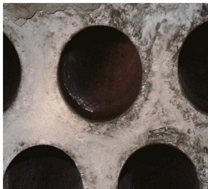
Clean boiler tubes provide optimal heat transfer leading to fewer gallons burned.
