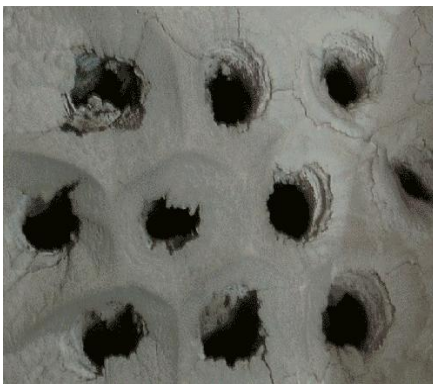
Burning No. 4 or No. 6 oil deposits layers of soot on the boiler tubes decreasing efficiency.
