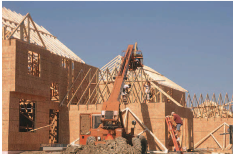
A strong ISR allows new construction and mitigates new pollution.
