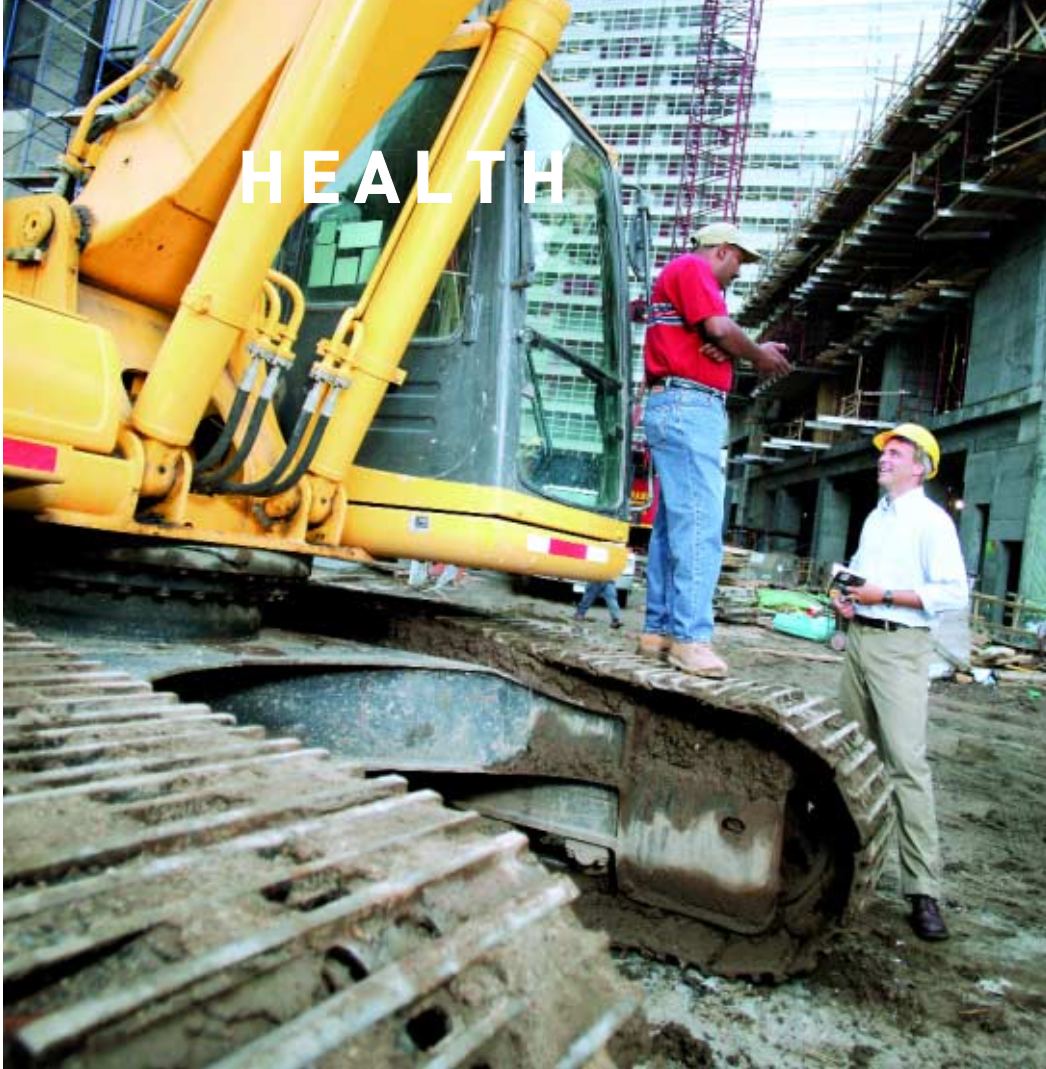
At ground zero, Andrew Darrell (right) talks with heavy equipment operator Hamid Kham. Nonroad diesel engines emit more harmful fine particles than all other mobile sources combined.
