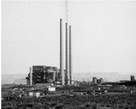
The Navajo power plant.
