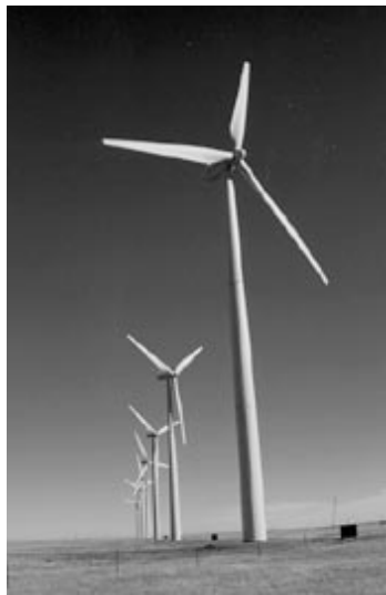
Colorado's Ponnequin wind farm makes "greener" electricity.
