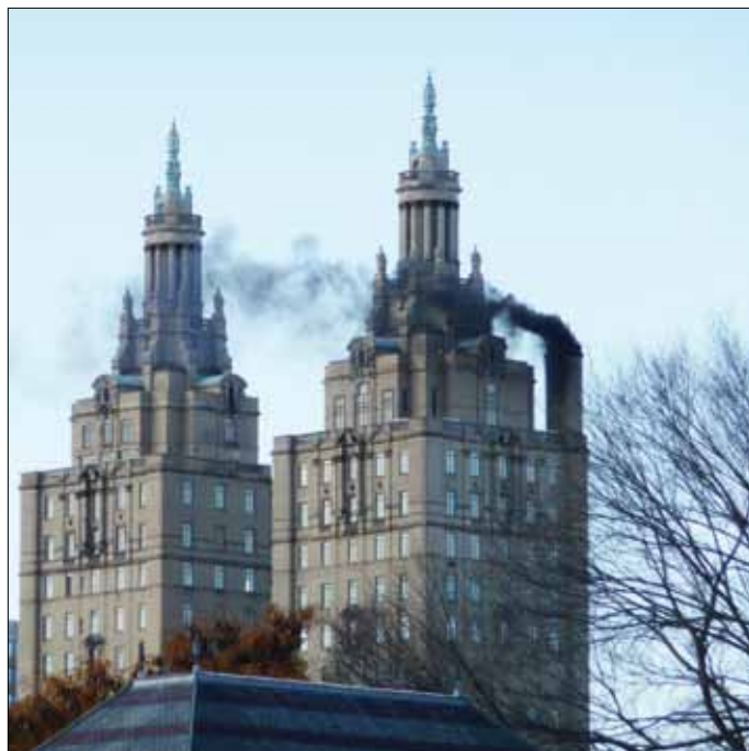
San Remo building burning No. 6 heating oil.
