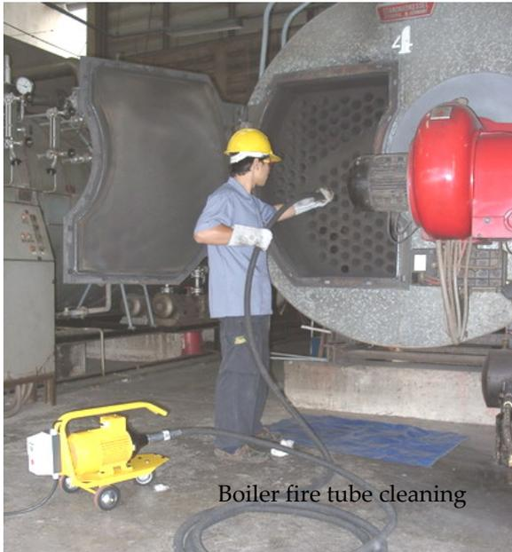
Boiler fire tube cleaning
