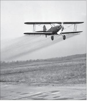
A specially equipped plane sprays DDT on a test site in 1947.
