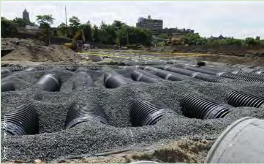
Underground stormwater recirculation tubes at Pier 6
