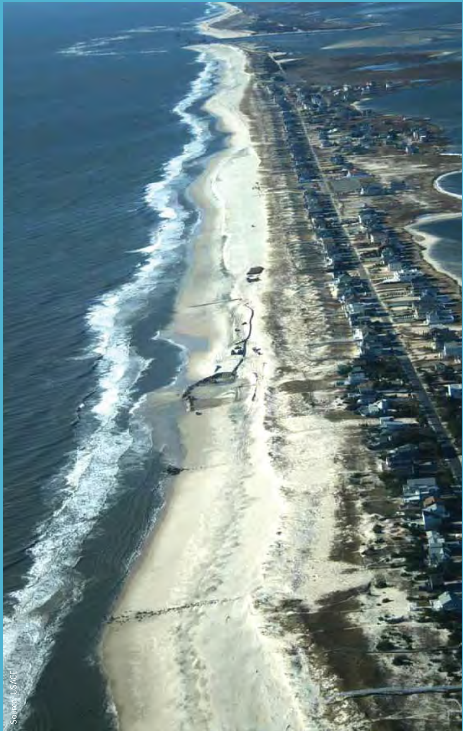
Groin 14 during re-nourishment in 2008 – vegetation in the background on the dune and berm
