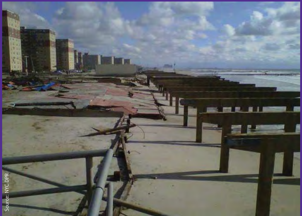
Rockaway Boardwalk, Queens after Sandy: Concrete pile sub-structure without wooden planking system
