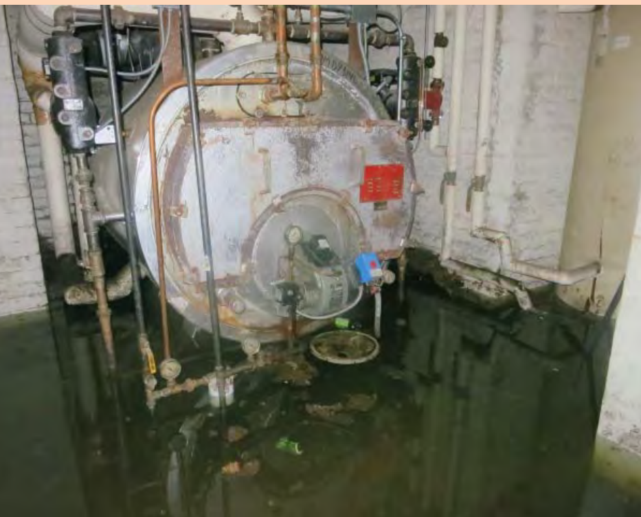
Flooded boiler
