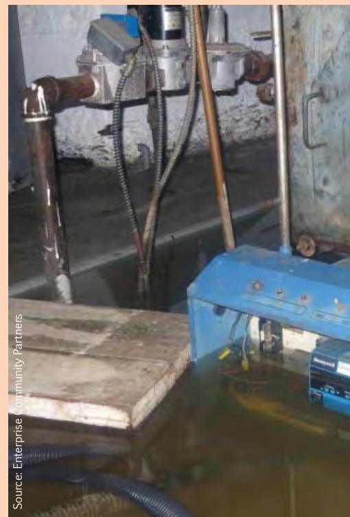
Flooded boiler
