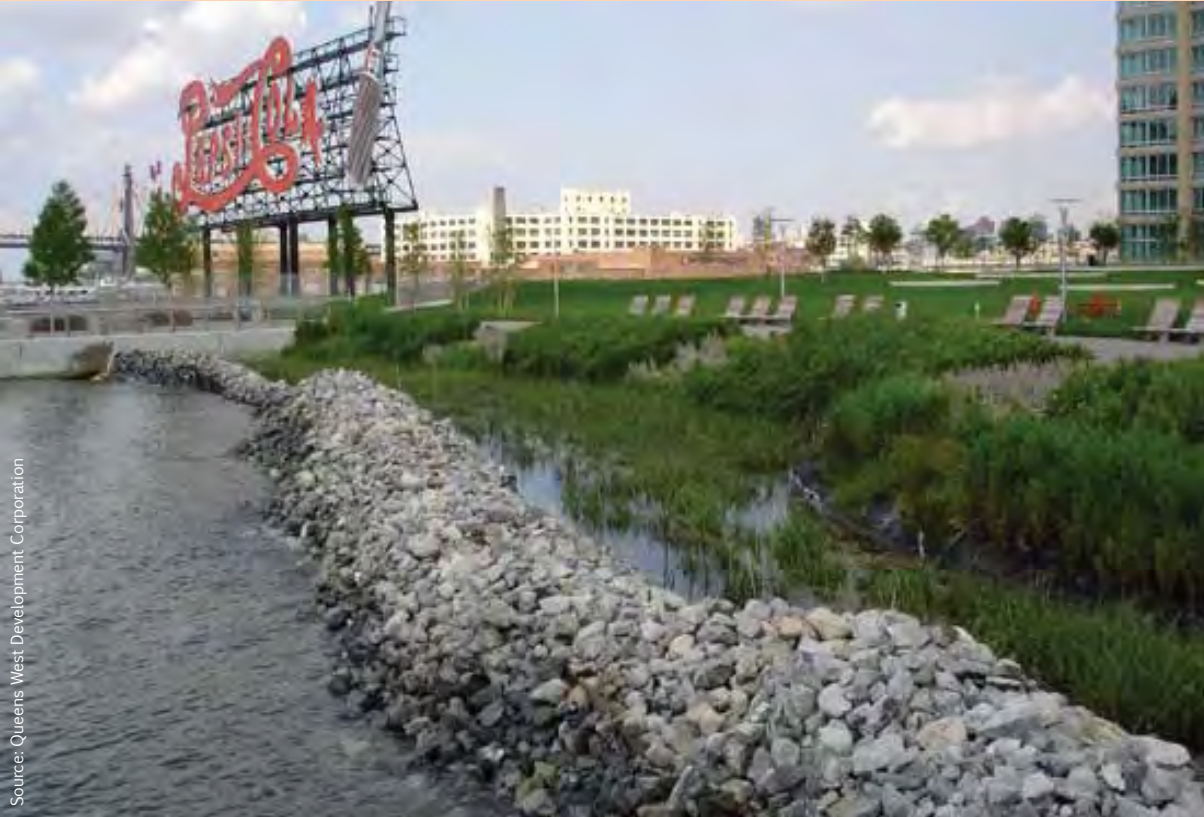
Rip rap along the water's edge at Gantry Plaza State Park
