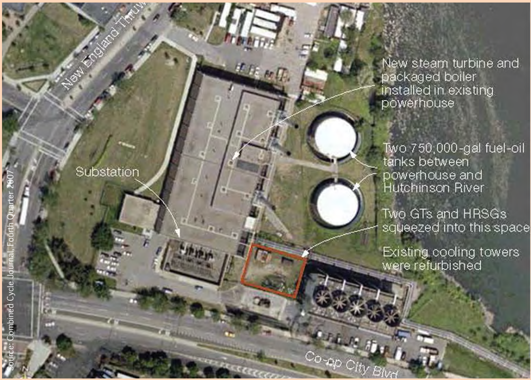
Co-op City's central plant and supporting structure
