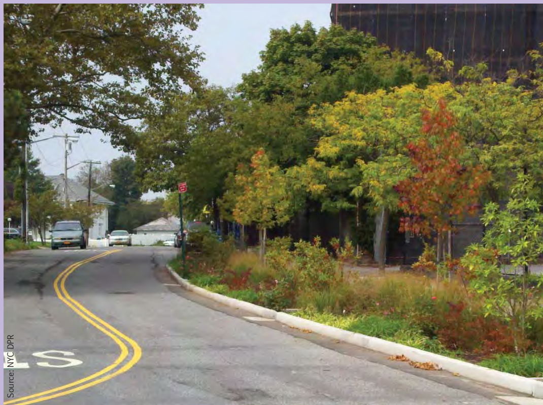
Installation along schoolyard to capture stormwater and encourage slower traffic at Westborne & Bay, Queens
