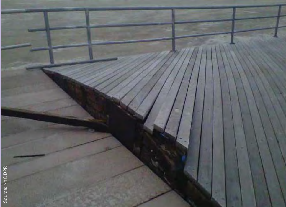
Destroyed hardwood decking besides pre-stressed concrete planking
