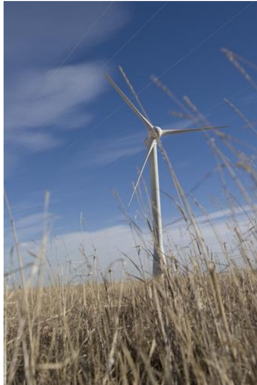
National Renewable Energy Laboratory
