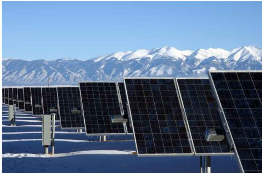
National Renewable Energy Laboratory
