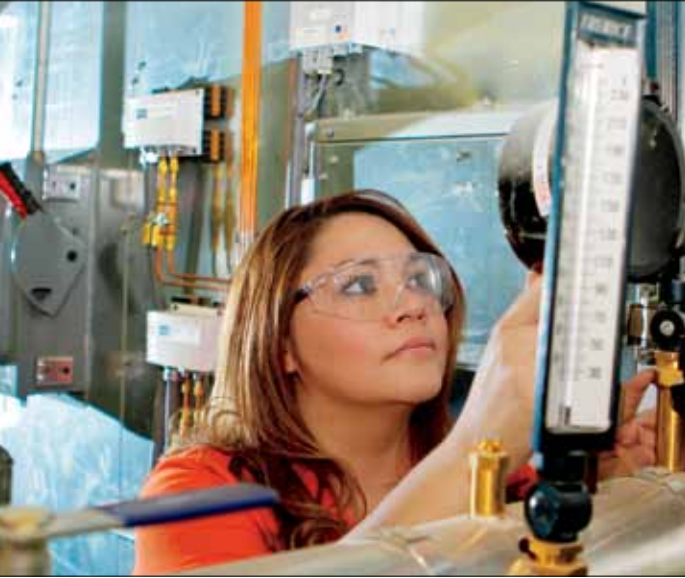
University of Texas at El Paso grad student Olivia Moreno studied building automation systems on campus during her EDF Climate Corps fellowship. Her recommendation to pre-cool buildings during off-peak hours will cut pollution.
