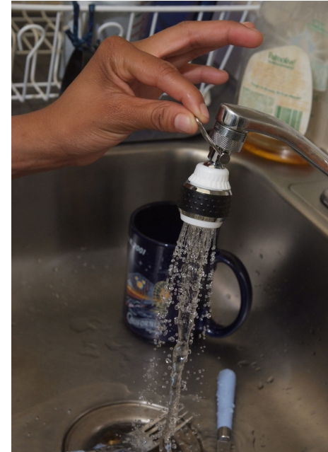
Simple devices like sink faucet aerators reduce water flows, save money, and avoid greenhouse gas emissions from treating, transporting and heating water.
