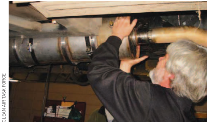
Installing a diesel particulate filter.
