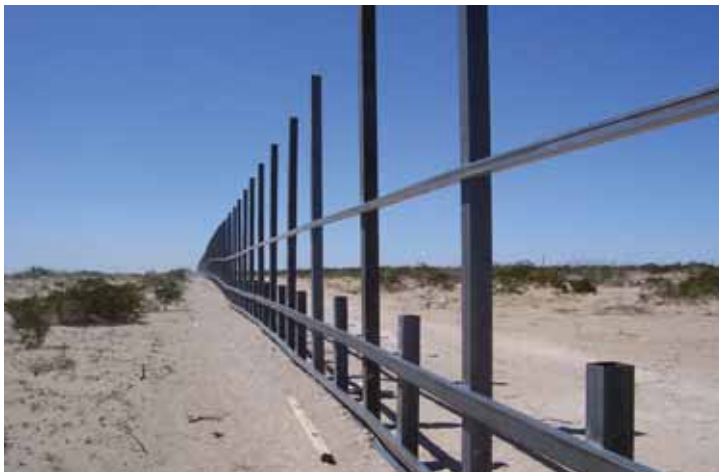
Under construction, the border fence.
