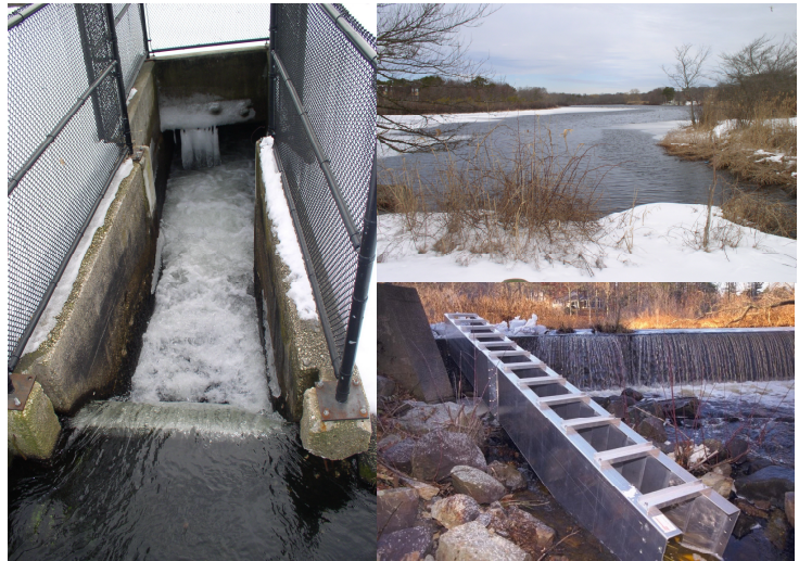
The narrow spillway at the Swan River dam in Brookhaven (left) prevents fish from reaching the large area of spawning habitat in Swan Lake (right, top). Installation of a fish ladder like this one from the Parker River in Massachusetts (right, bottom) can allow fish to swim past this obstacle. (ladder photo from NOAA)
