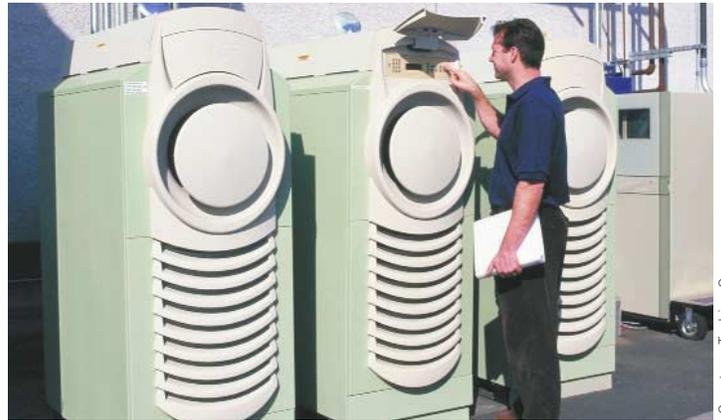
New microturbine generators produce less pollution without diesel.
