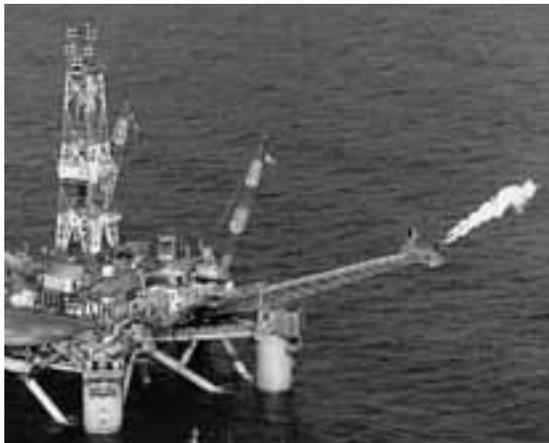
One of the steps BP will take to reduce greenhouse gas emissions is to curb the "flaring" or burning off of waste gas, as seen above from this platform in the North Sea.
