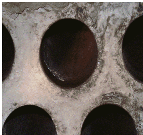
Picture showing clean boiler fire tubes
