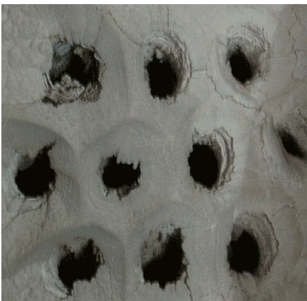
Picture showing dirty boiler fire tubes
