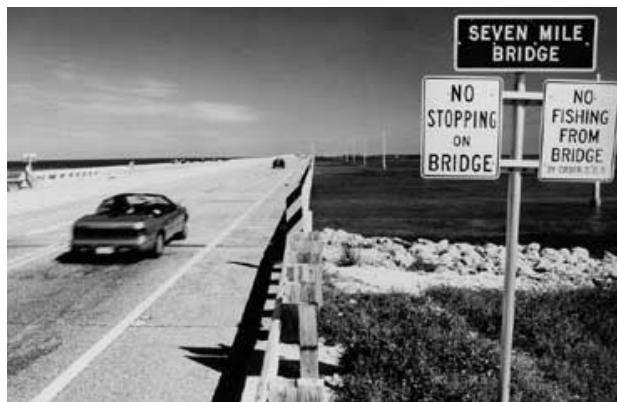
Widening U.S. Route 1 between the Florida Keys and the mainland would have harmed wetlands and an adjacent coral reef.
